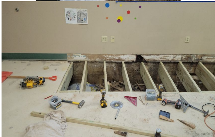
Classroom Floor Repair
