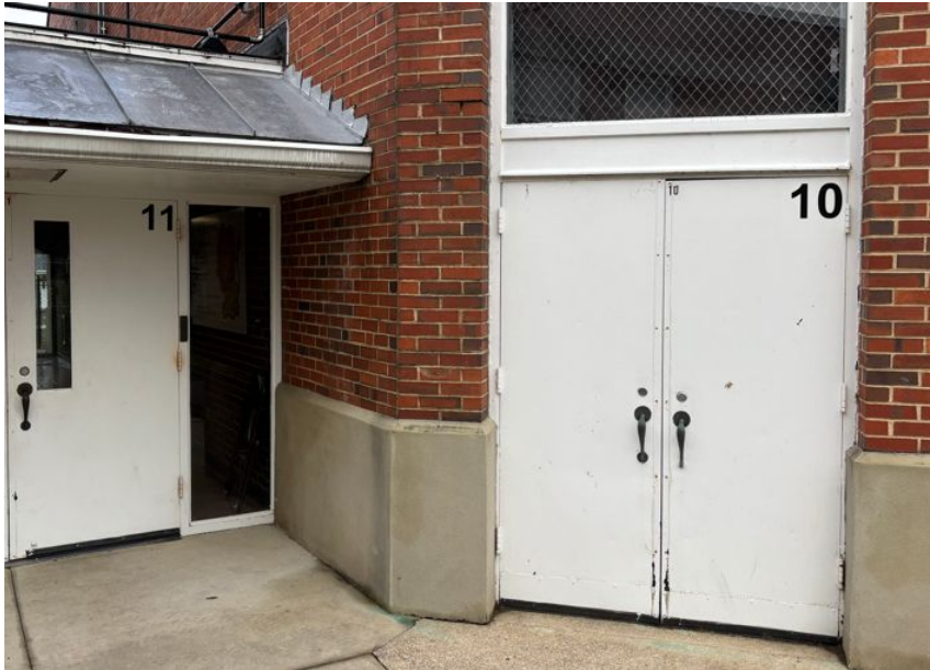
Numbered All Exterior Doors – System Wide
