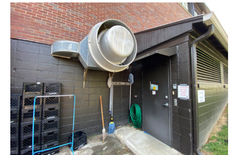
08 Fan unit is exposed and within public view
