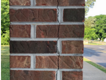
01 cracking brick
