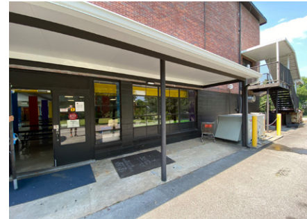
03 exterior finishes showing normal wear
