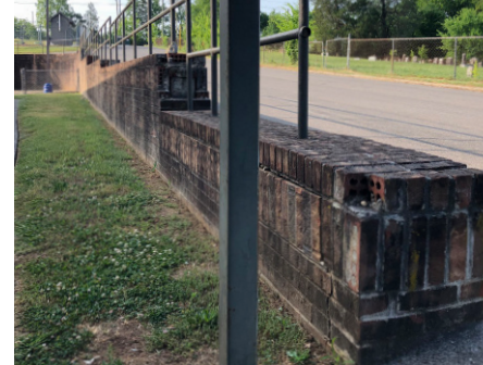
03 masonry deterioration
