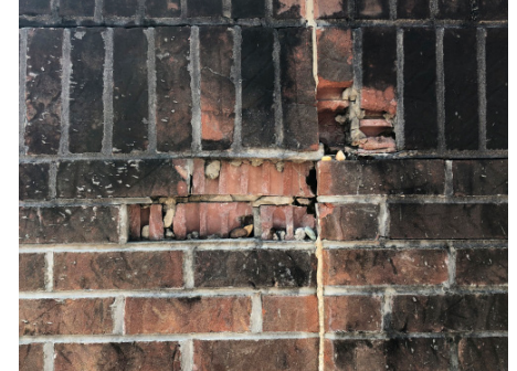
04 masonry deterioration
