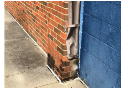
08 damaged downspout
