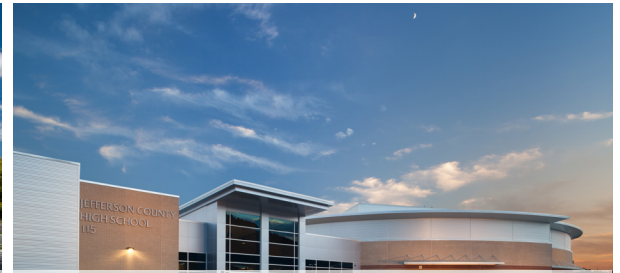
JEFFERSON COUNTY HIGH SCHOOL
