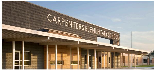
CARPENTERS ELEMENTARY SCHOOL
