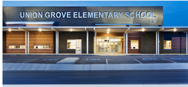
UNION GROVE ELEMENTARY SCHOOL
