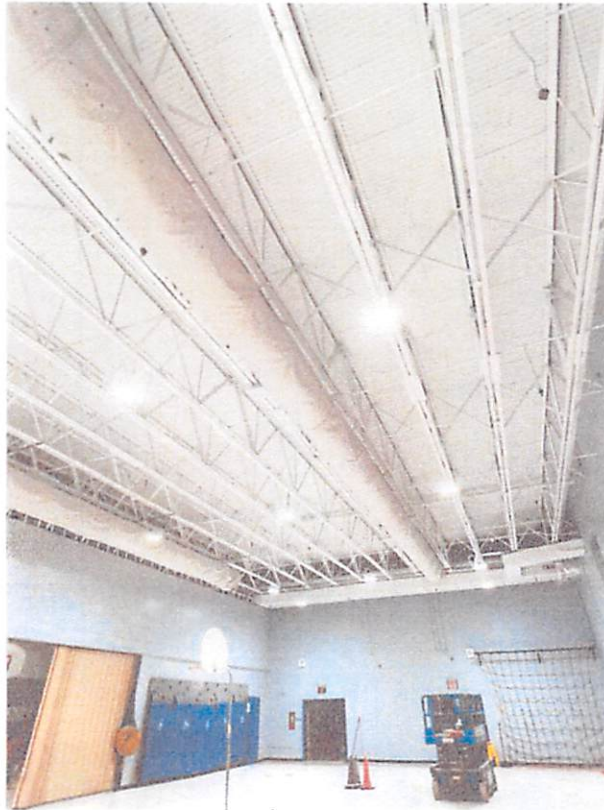
Westhills Elementary-gym ceiling June 30, 2023
